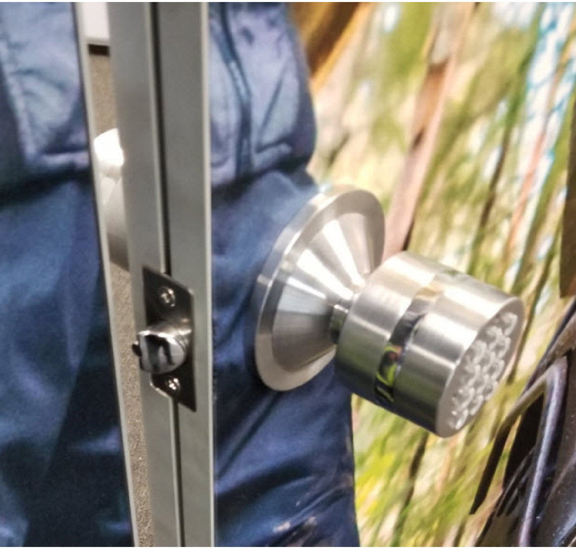
Uninstall the Handle Latch.
